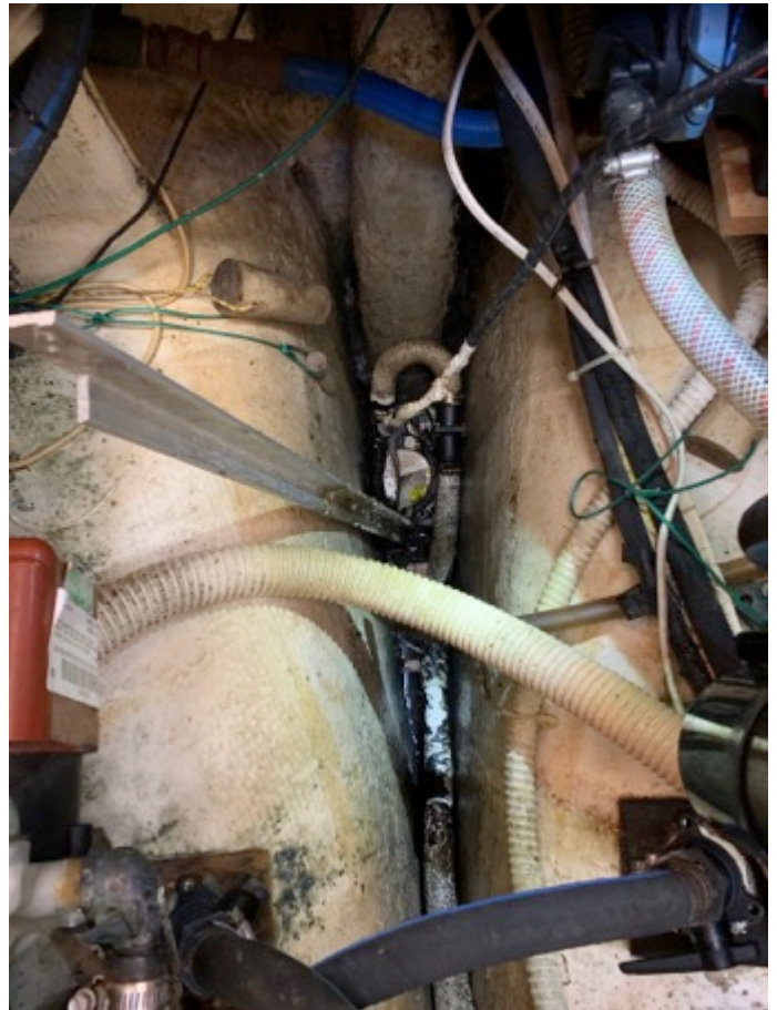
Deep bilge; black oily residue at the bottom
