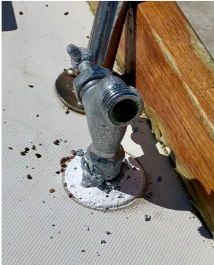
Deteriorated deck wash spigot thru deck fitting
